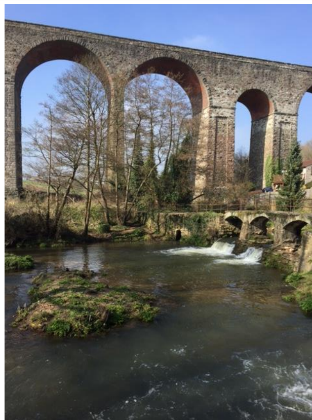
3 – Pensford Viaduct and the Weir
